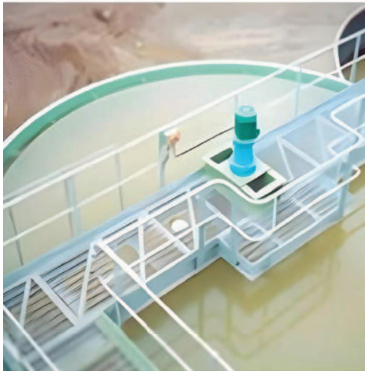
High Rate Solid Contact clarifier (HRSCC)
